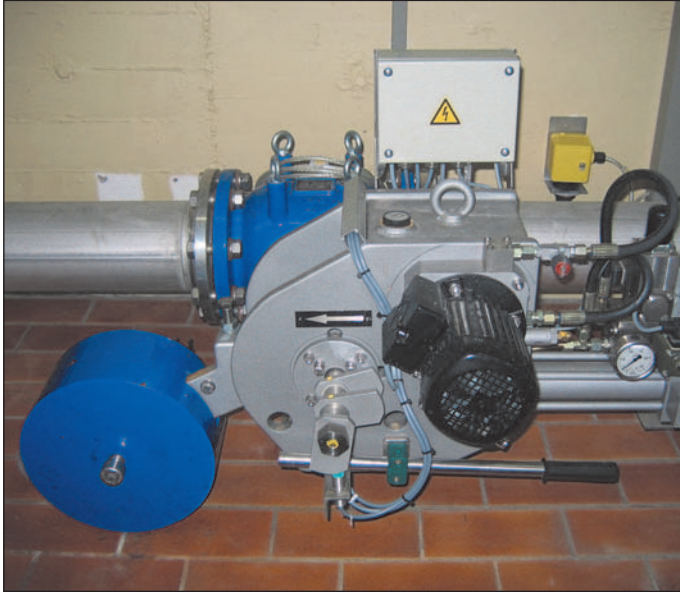
Horizontal cylinder, anti clockwise closing VAG RIKO® Plunger Valve DN 150 with Brake-and-Lift Cylinder, installed in the pumping station in Neuenkleussheim in Germany.
